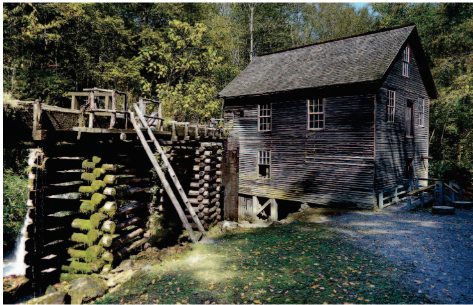
Park It Forward revenues will allow the park to tackle rehabilitation work at Mingus Mill, a historic gristmill built in 1886.
