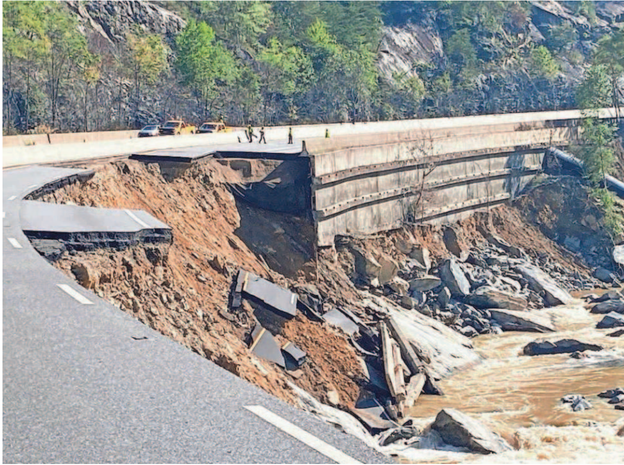
A 4.5-mile section of I-40 in the Pigeon River Gorge was destroyed during Tropical Storm Helene. There is no reopening date set. PROVIDED BY NCDOT
