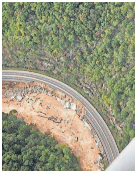
Extreme erosion tore up the highway and destabilized the slope for miles along I-40 through the Pigeon River Gorge. PROVIDED BY NCDOT
