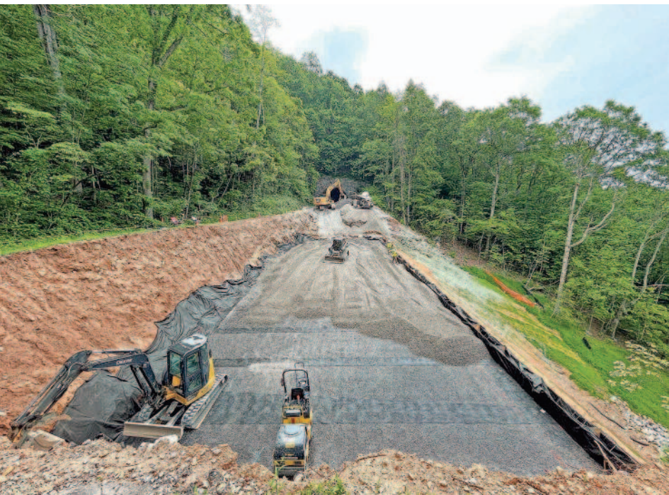
National Park Service repair crews have begun repairing a landslide at Milepost 401 near Ferrin Knob Tunnel #3. PROVIDED BY NATIONAL PARK SERVICE
