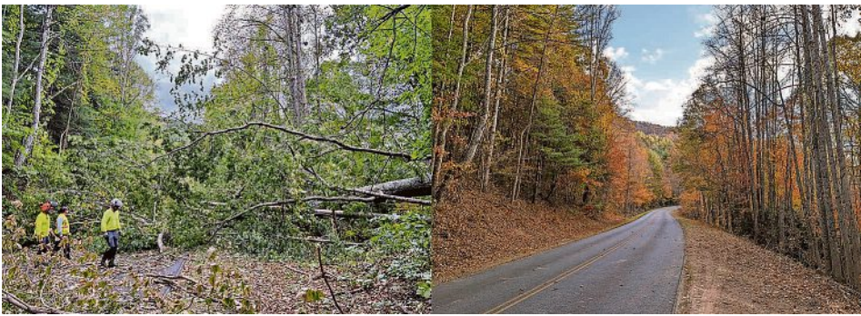
Tropical Storm Helene left this section of the Blue Ridge Parkway near Asheville completely blocked by fallen trees, at left. Crews were able to clear it within six weeks of the storm, though many other sections remained closed for much longer, and some have yet to reopen. RIGHT PHOTO BY J. SHAFER, BOTH PROVIDED BY OF NPS
